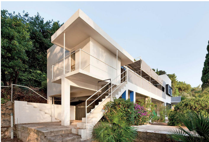
WHITE HOUSE | The restoration of Eileen Gray's E.1027, photographed above in 2010, began over decade ago. Among other problems, some of the original features were replaced with inferior materials. © MANUEL BOUGOT
